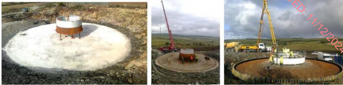
Figure 2.6 Wind Turbine Foundation Formation, Steel Reinforcement and Concrete Pour (Source: Mable Consulting Engineers)
